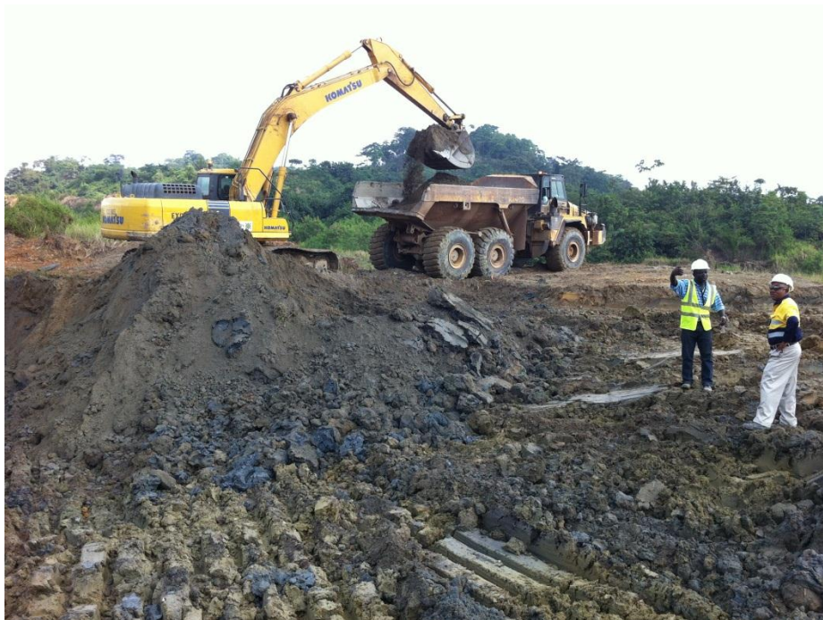
Reclaiming Tails in Dam 1
