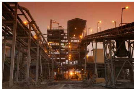
Processing plant & conveyor belts before the refurbishment Source: Company
