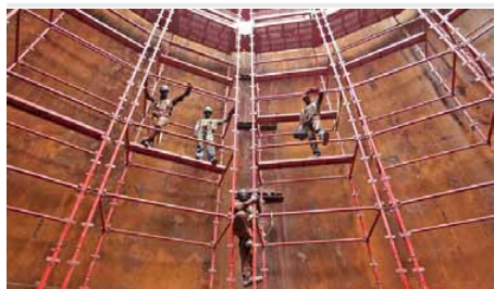
Refurbishing the CIL tanks Source: Company Presentation
