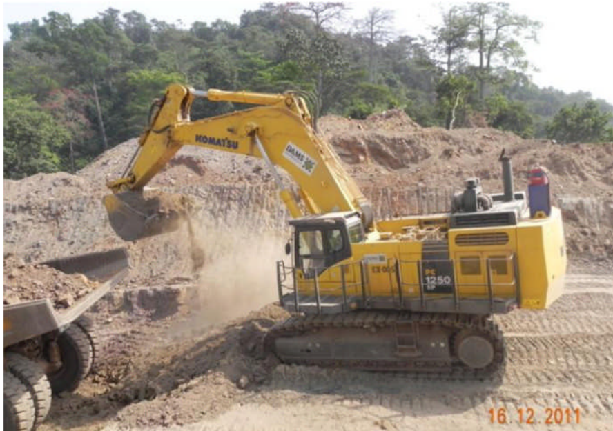
Noble's 125 ton excavator at work
