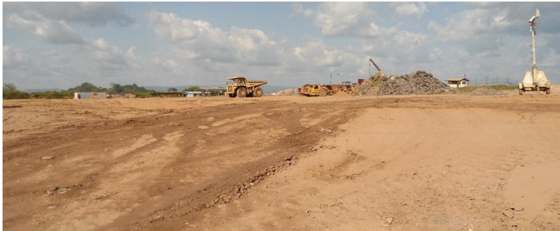
ROM pad extension
