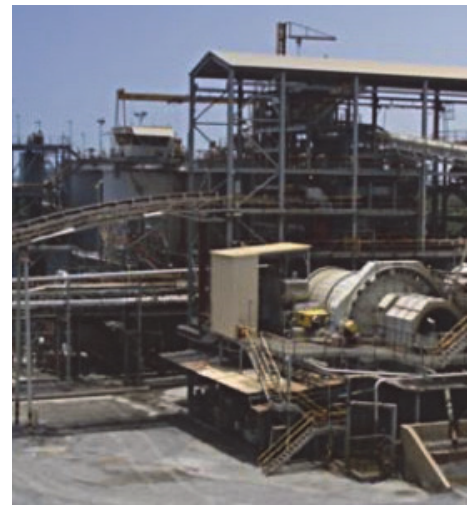
Figure 13: Bibiani CIL Processing Plant
