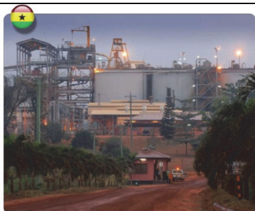
Figure1: Bibiani's Processing Plant
