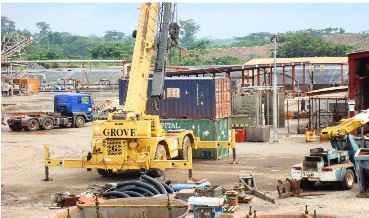
Crane loading supplies at processing plant
